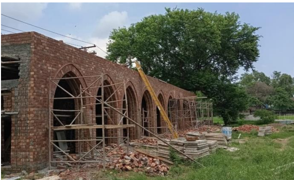
Rehabilitation Centre & Café Construction Hill Lahore, Diocese Sargodha Rs. 18.11 Million
